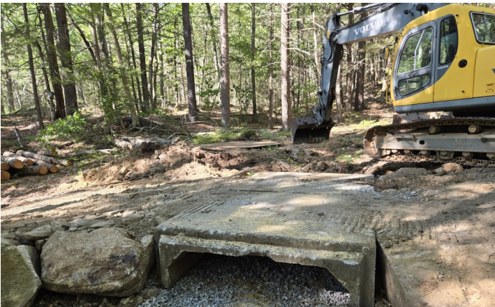
The Red Cross-Over Trail has had culverts and ditching added along the trail to handle water drainage.
