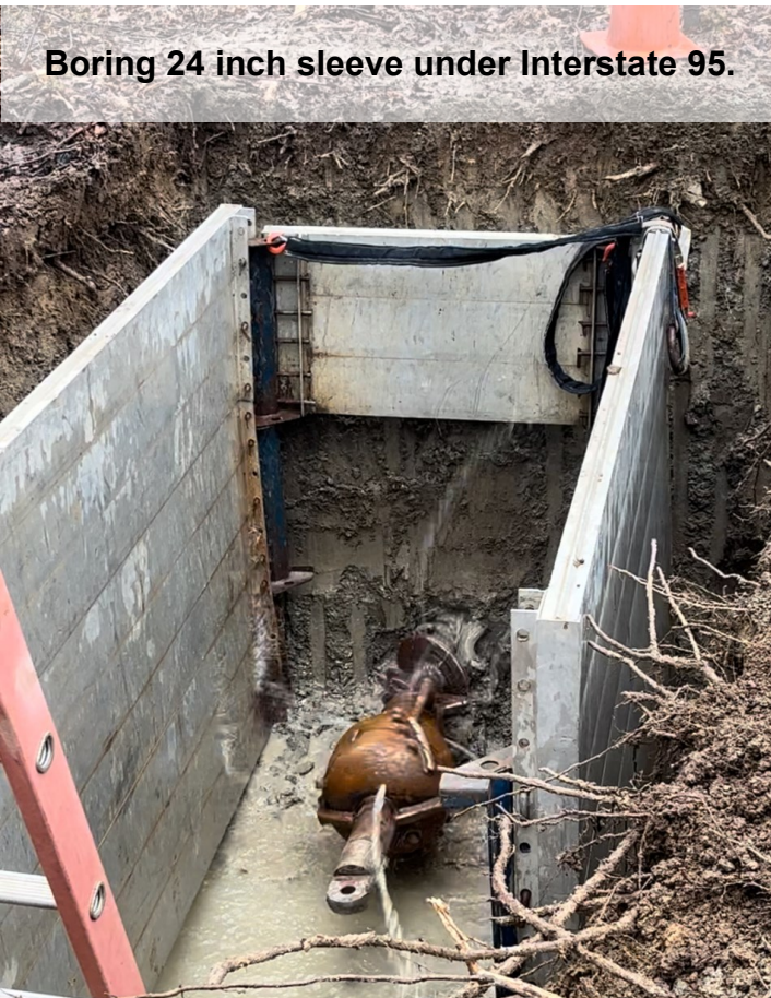
HDPE pipe inserted into sleeve beneath Interstate 95.
