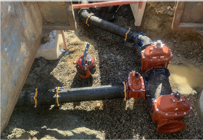
Three-way valving at the intersection of Lindsay Road and Loving Kindness Way.
