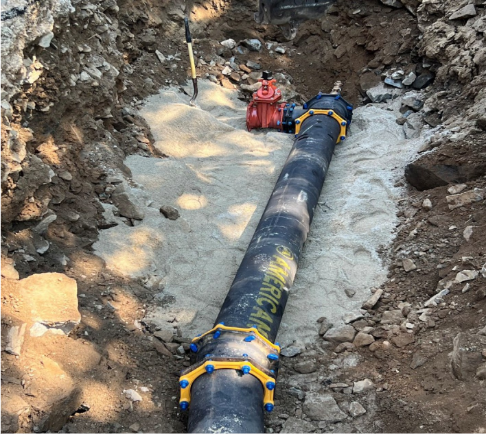
A ten-inch main extension and six-inch service at 1132 US Route One.
