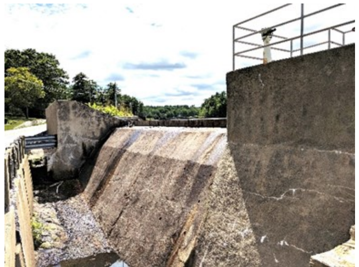
Last month, operators opened the dam release gate to bypass more water into the stream .
