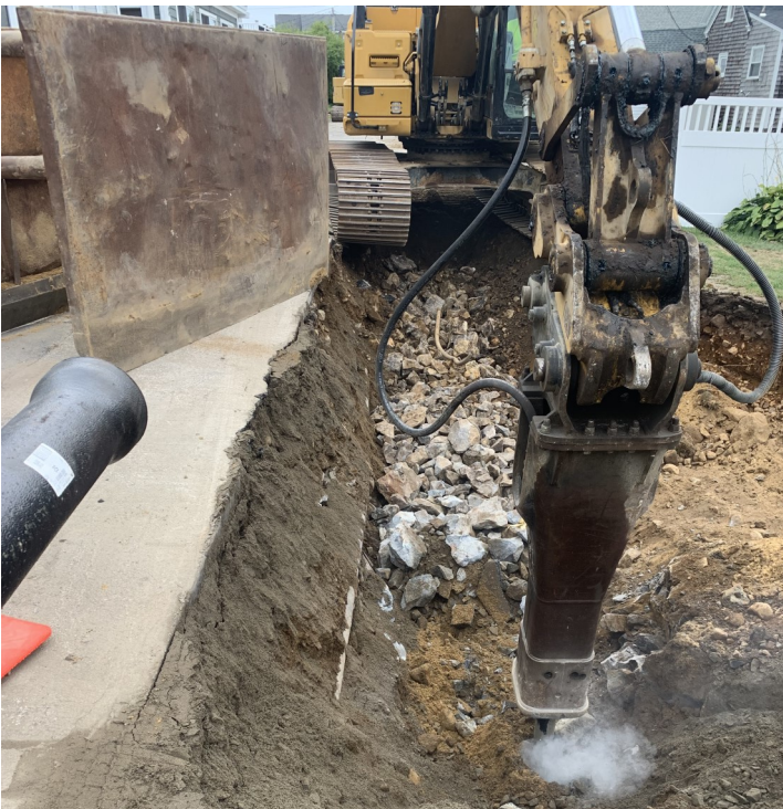
Hammering hard ledge on High Street
