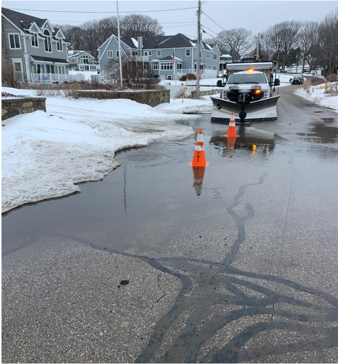
Leak on Norton Farms Road
