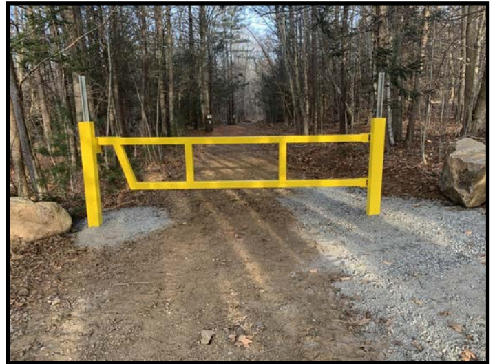
Replacement gate at the transmission main access road in the Whippoorwill subdivision. A similar gate was installed at the Simpson Hill Tank access road.
