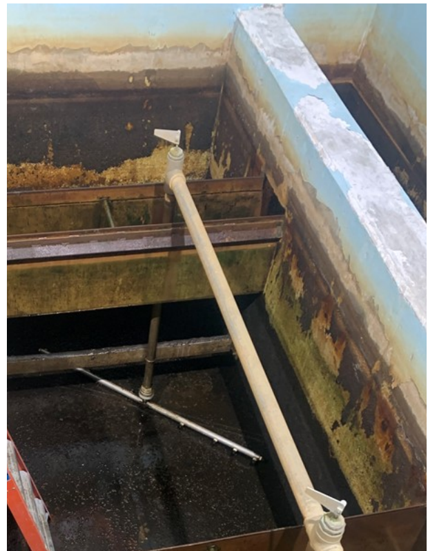
Surface Wash Arm Nozzle Repair
