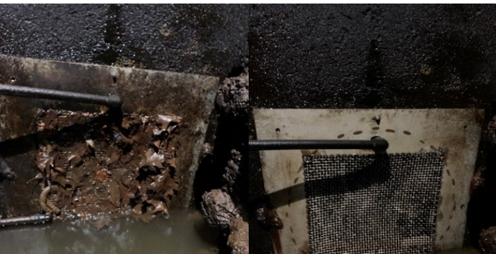
Secondary eel & debris screen cleaning, before entering the pipe to the plant .
