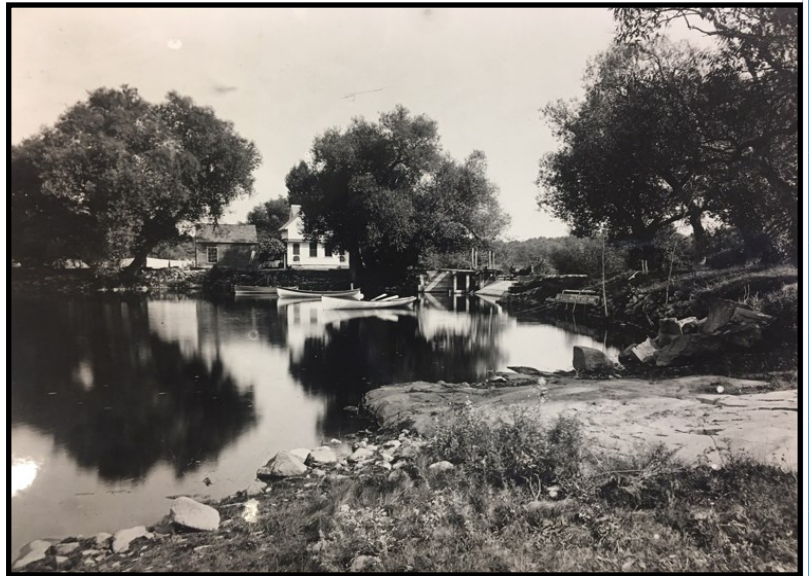
Chases Pond Dam. Early 1900's
