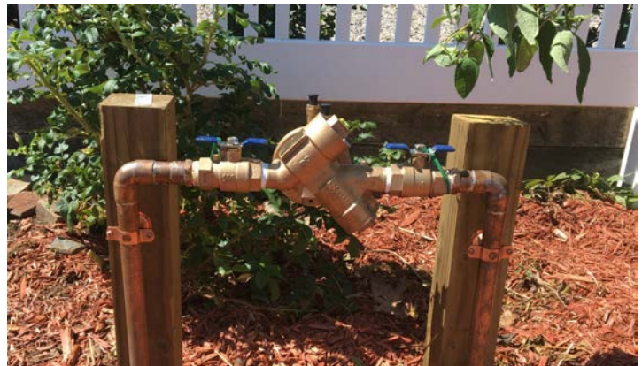
Backflow Prevention Device
