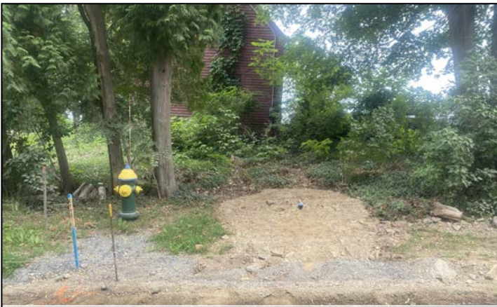
Future one-inch water service for 230 Southside Road
