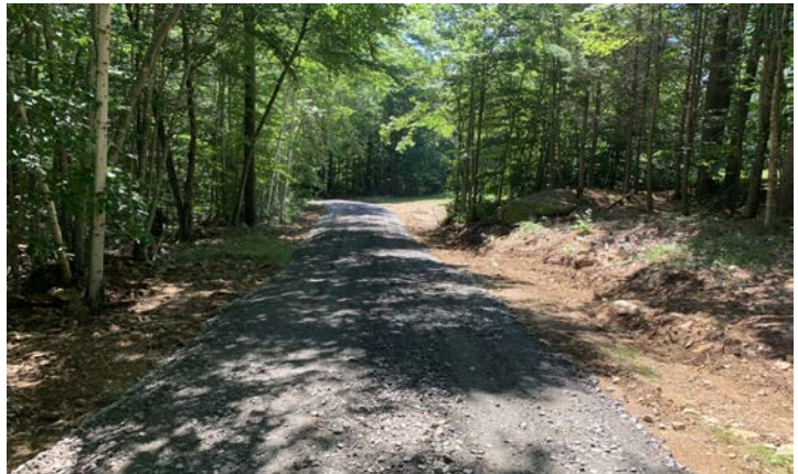
New gravel and ditching on the Red Management Road.
