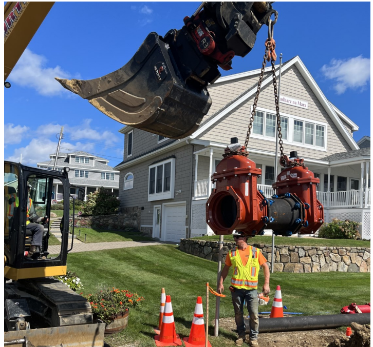
Curtis Earthworks has completed the Nubble Road Phase III main replacement project.
