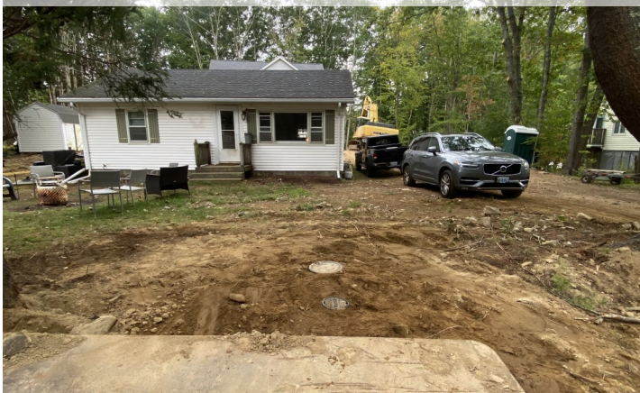
A homeowner financed water main extension was installed on Rogers Road.
