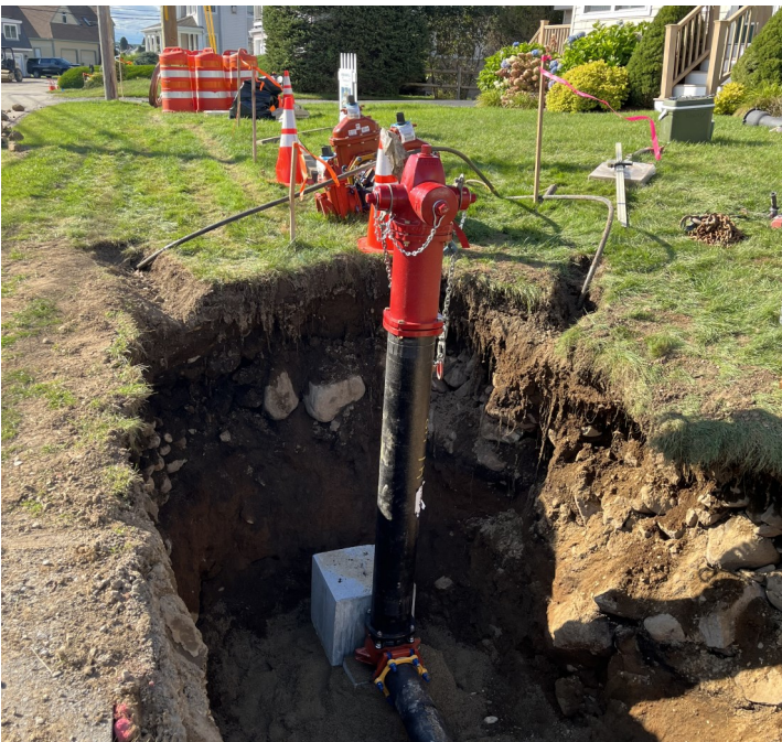
New fire hydrant on the corner of Fourth Avenue and Nubble Road.
