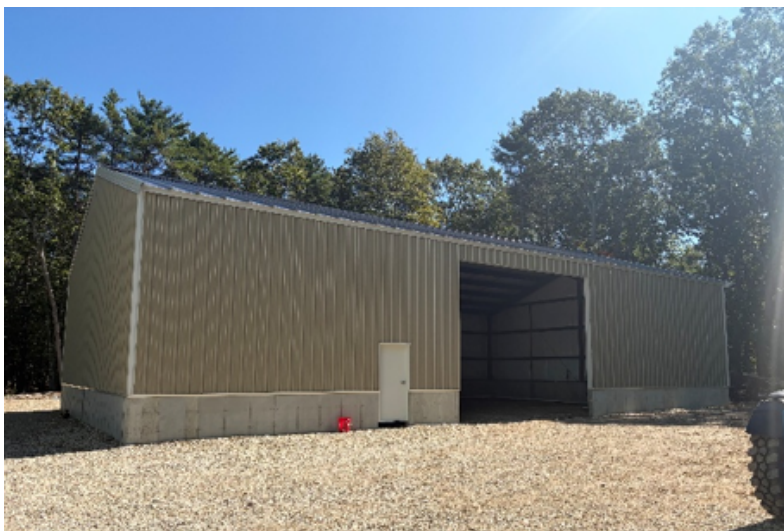
Completed Simpson Hill Tank Storage Building
