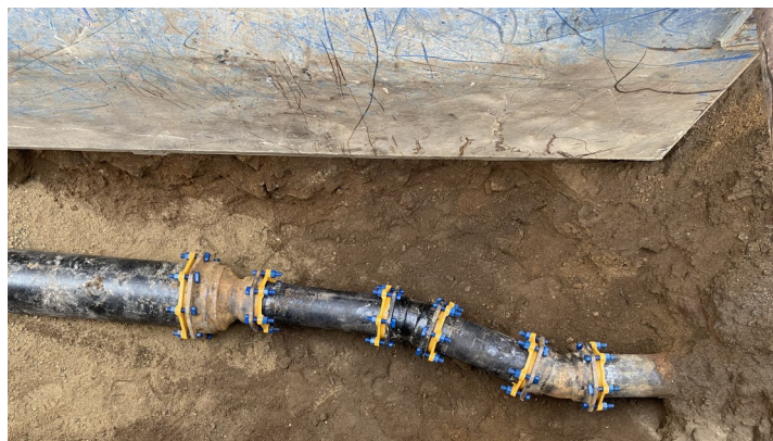
Final connection of ten-inch to the six-inch main on Nubble Road.
