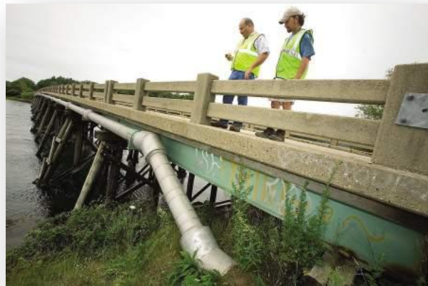
Don Neumann, left, supervisor of the York Water District, and Todd Hill, right, the coordinator of the geographical information systems in York, show how the existing water line, shown in metal insulating cover and currently afixed to the Route 103 bridge over the York River, will be moved about 60 feet under the river as the bridge is being repaired by Maine DOT
